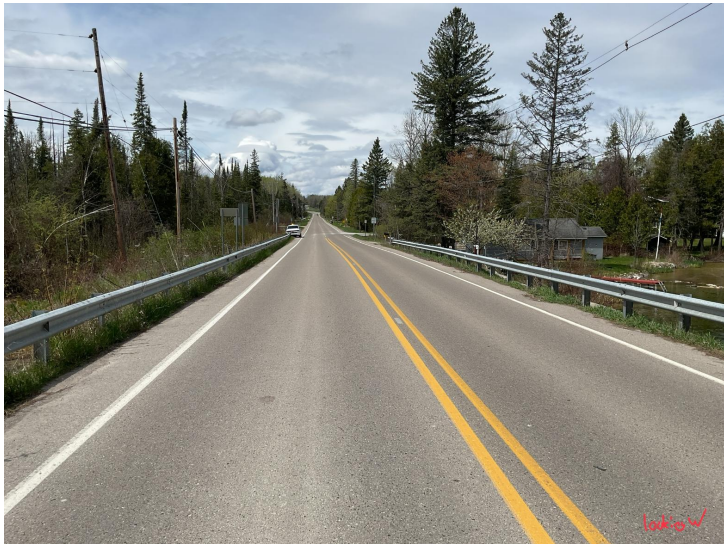
Document Name: IMG_0174.JPG Category: Approach Span Number: Comments: Looking west
