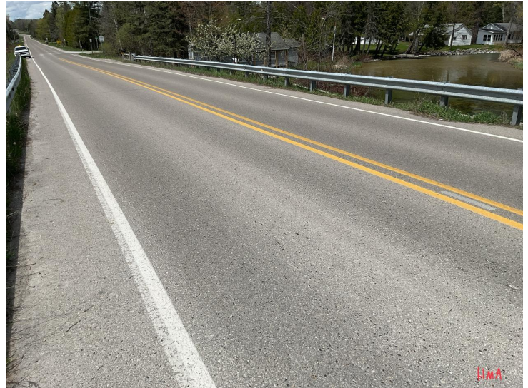
Document Name: IMG_0175.JPG Category: Deck Span Number: Comments: HMA surface
