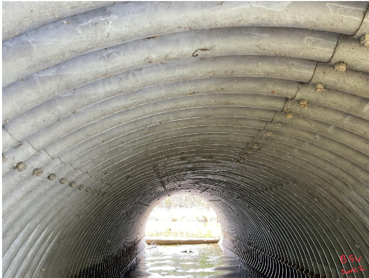
Document Name: IMG_0195.JPG Category: Culvert Span Number: Comments: Barrel 5W, soffit
