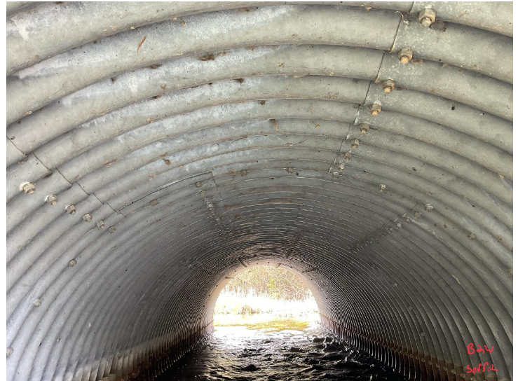
Document Name: IMG_0186.JPG Category: Culvert Span Number: Comments: Barrel 2W, soffit
