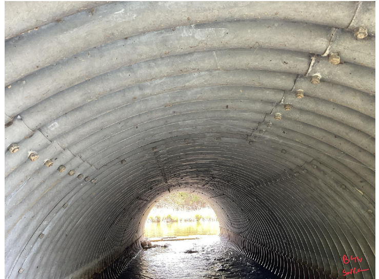
Document Name: IMG_0192.JPG Category: Culvert Span Number: Comments: Barrel 4W, soffit
