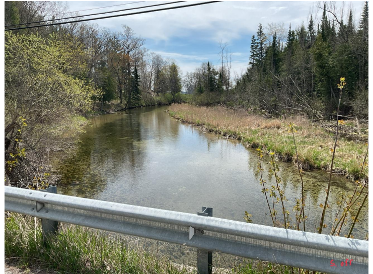
Document Name: IMG_0177.JPG Category: Channel Span Number: Comments: South channel
