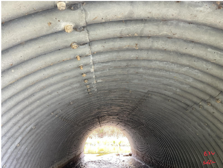
Document Name: IMG_0189.JPG Category: Culvert Span Number: Comments: Barrel 3W, soffit
