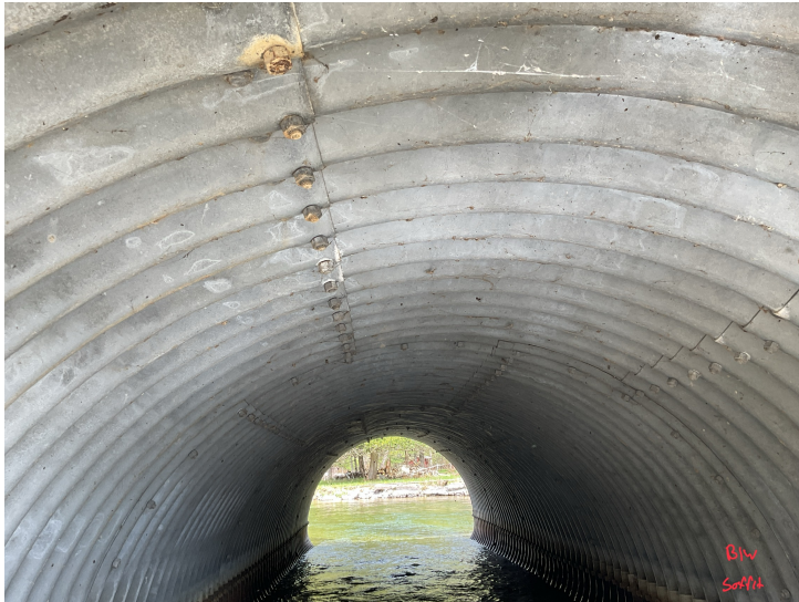
Document Name: IMG_0183.JPG Category: Culvert Span Number: Comments: Barrel 1W, soffit
