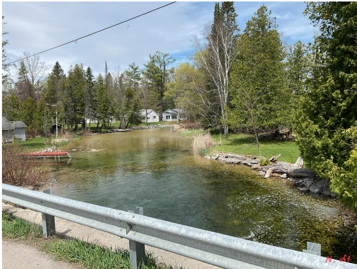
Document Name: IMG_0179.JPG Category: Channel Span Number: Comments: North channel
