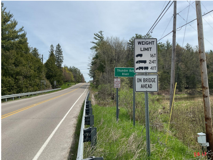
Document Name: IMG_0172.JPG Category: Posting Span Number: Comments: EB load posting
