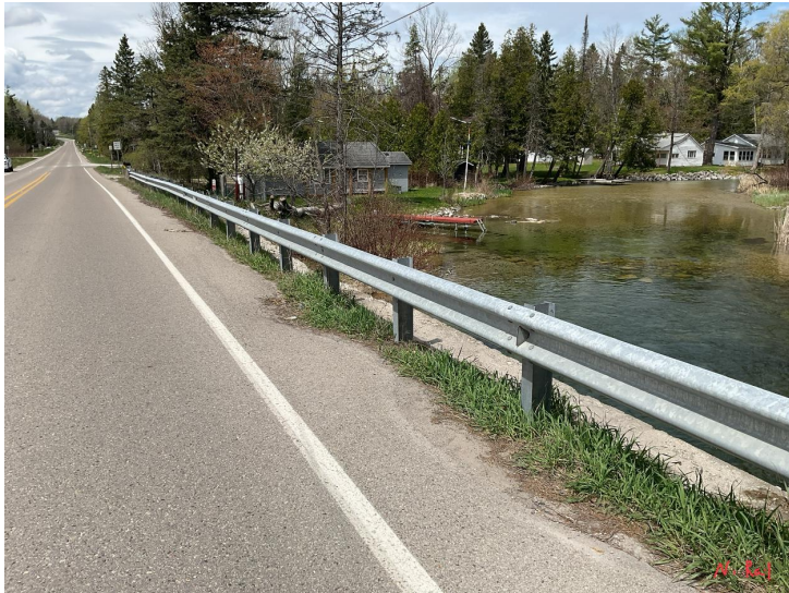
Document Name: IMG_0178.JPG Category: Railing Span Number: Comments: North rail
