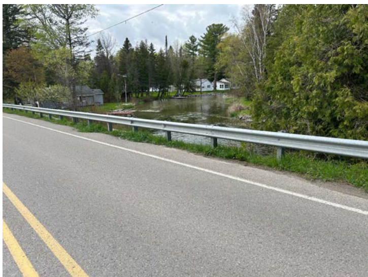
Document Name: IMG_5685 conv.jpeg Category: Railing Span Number: Comments: N rail
