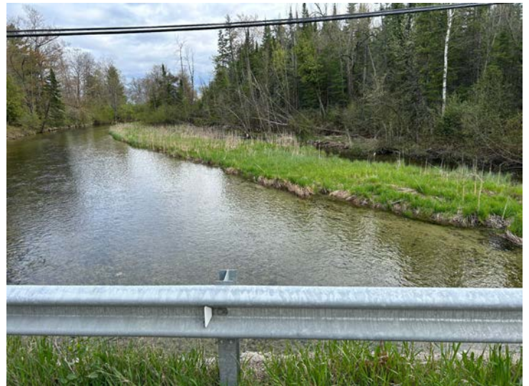
Document Name: IMG_5686 conv.jpeg Category: Elevation Span Number: Comments: Looking S off structure
